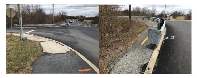
Status: No decision on project or funding source yet. Removal of guardrail, installation of an ADA-compliant curb cut, and an improved trail surface are needed at the intersection.
